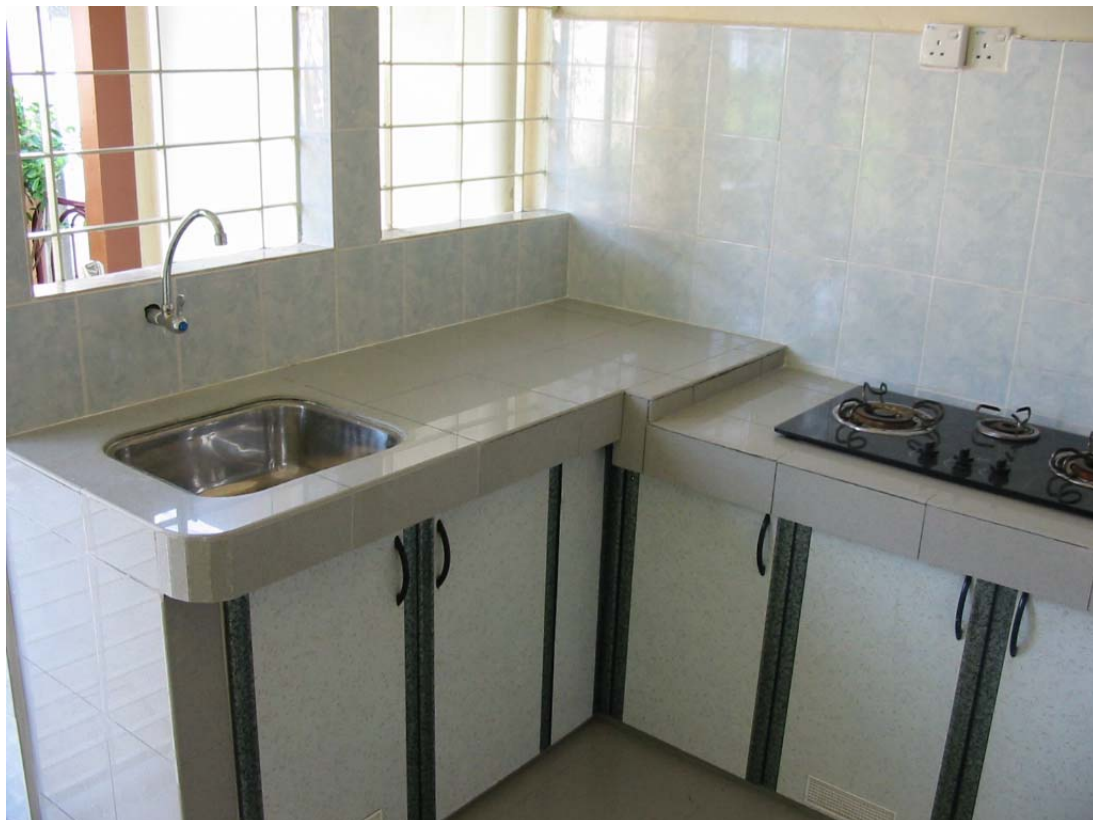
Single sink and extended tiled worktop in wet kitchen with built-in 3-burner stove.
