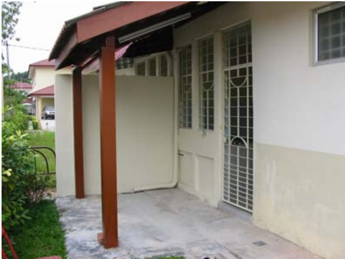
Extended rear verandah with lighting and cement floor
